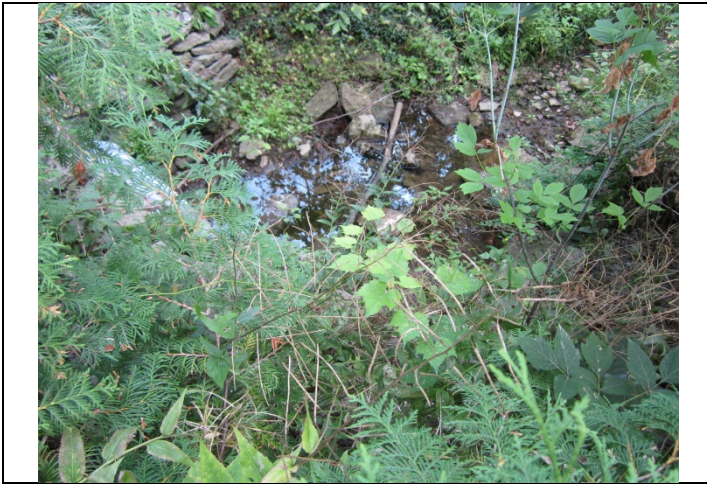
Photo 18 Station 55 – upstream view from Front Road showing channel overview.
