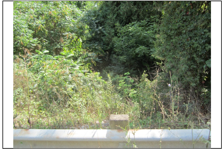
Photo 19 Station 57 – facing upstream from Front Road showing channel overview
