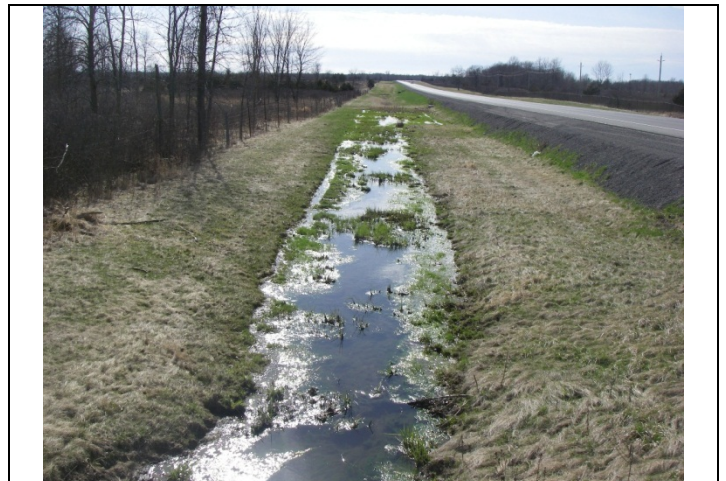
Photo 12 M9 – Facing downstream along Taylor Kidd Boulevard showing channel overview.
