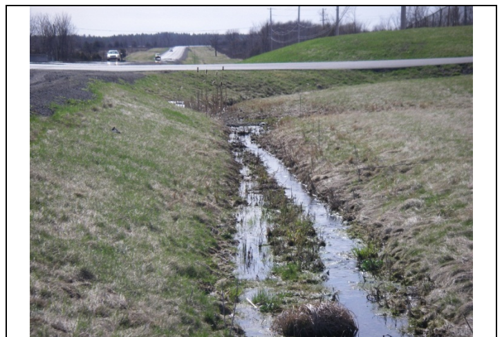
Photo 10 M4 – Facing downstream along Taylor Kidd Boulevard showing shallow channel.
