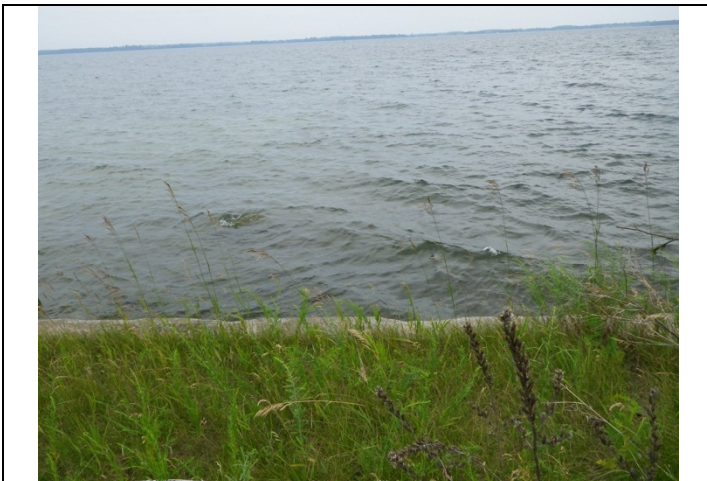
Photo 5 M2 – Facing downstream showing culvert and direct connection to Lake Ontario.
