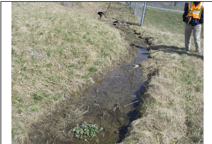
Photo 17 M10 – Facing upstream showing channel overview and possible patch of watercress.
