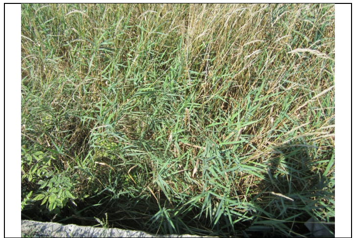
Photo 4 Station 58 – Close-up of culvert and dry channel.
