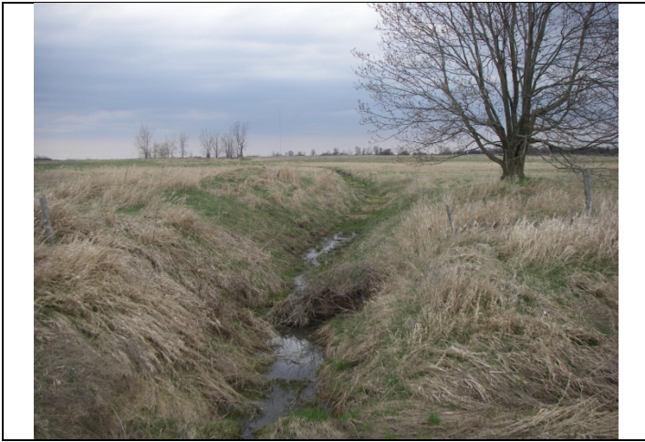
Photo 25 Station 53 – Upstream view from 2 nd Concession showing channel overview.
